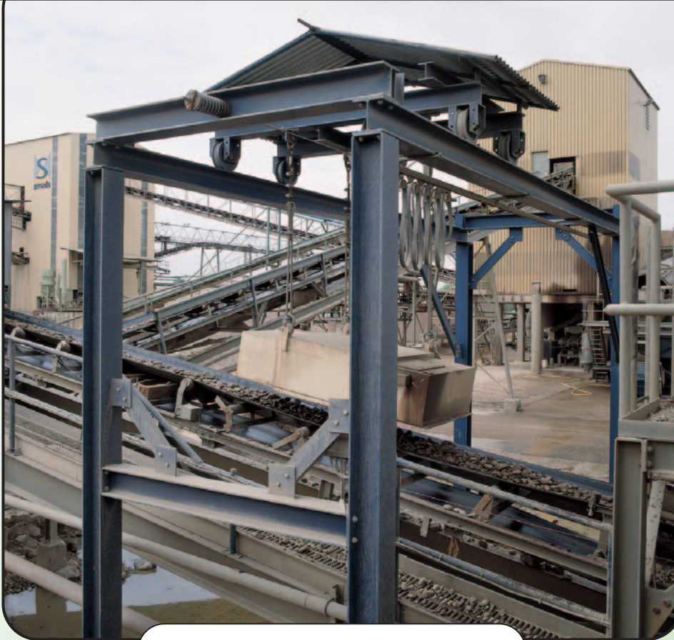
Electro block magnet (5.5 kW, for deferrisation of gravel.
