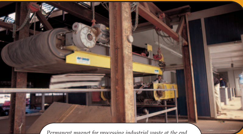
Permanent magnet for processing industrial waste at the end of a grading line. Installation in-line above belt.
