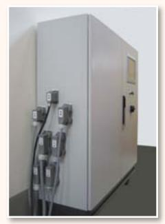
Cable connection between control panel and I-Sens is afffected by means of connectors.
